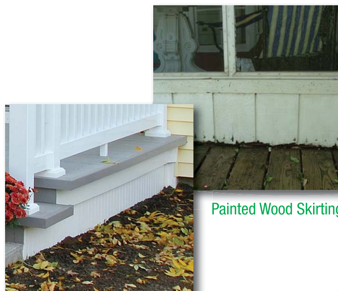
PVC Bead Board Used as Skirting at Building Grade
